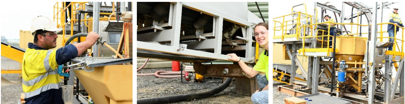
Figure 1: JTMS staff commissioning the plant.
