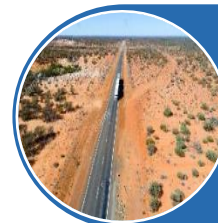
Goldfields Highway (access to Geraldton port)
