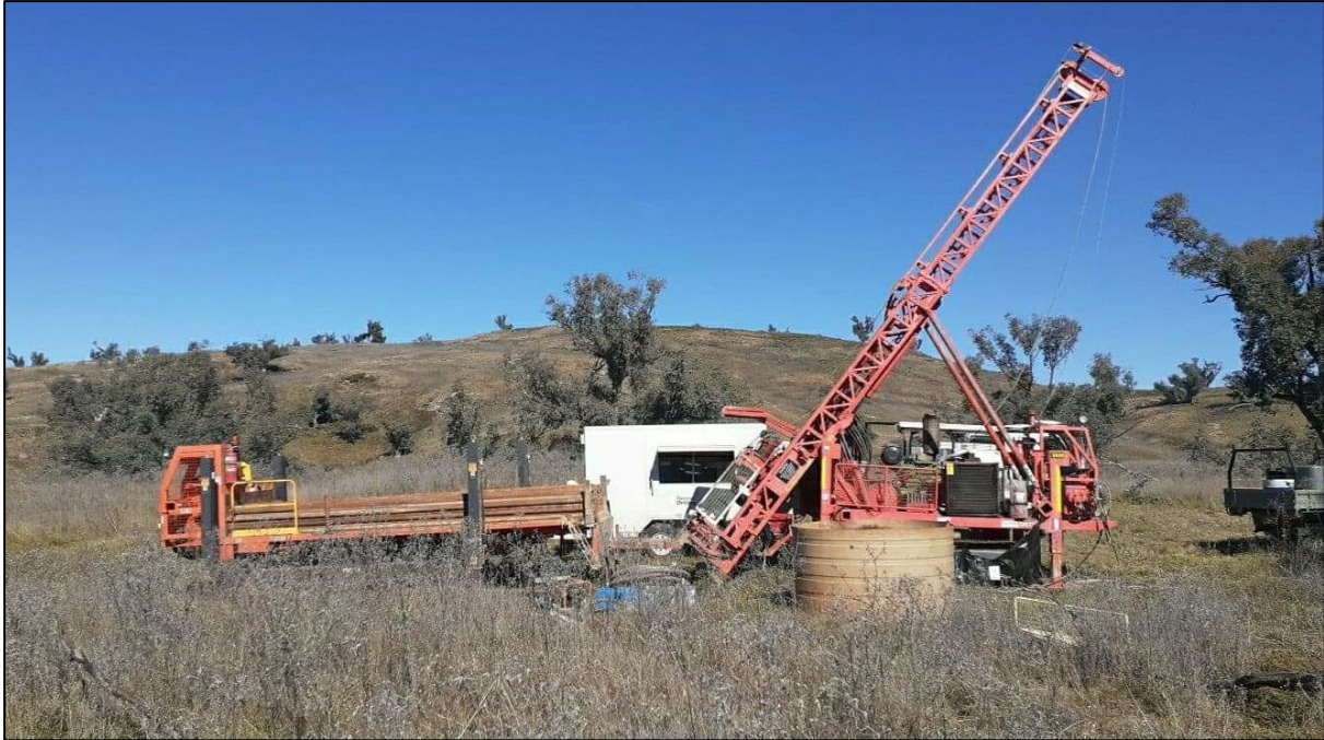
Figure 1: Diamond drill rig setting up over Hole 1 at Big Hill
