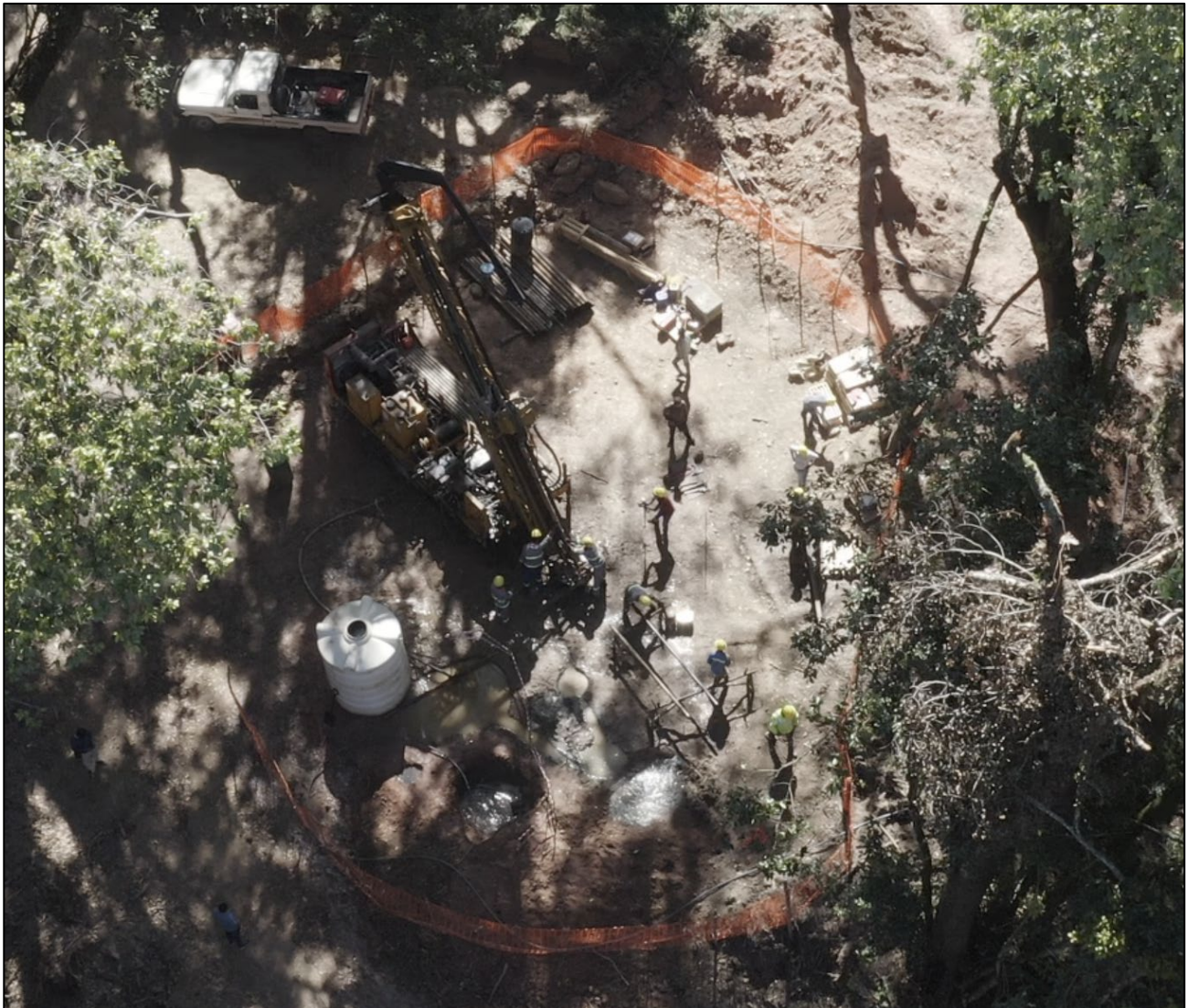
Figure 5 – Megado's team working the first drillhole at the Babicho Gold Project
