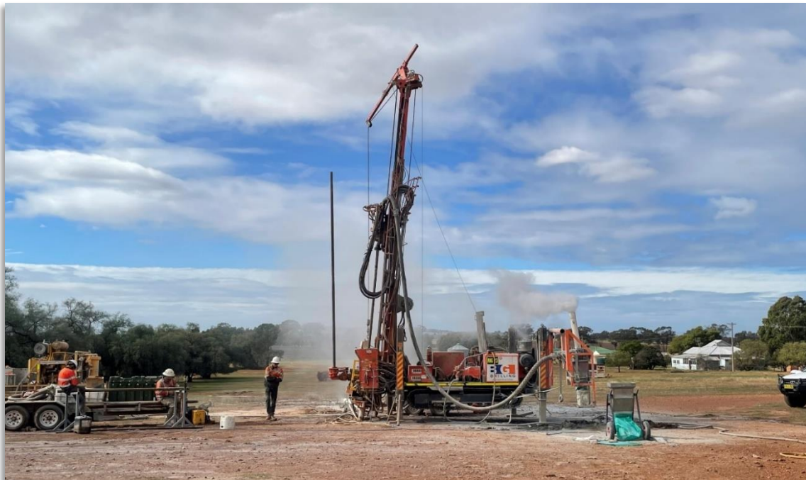
Figure 1: Drilling RC hole KBRC007 at Goodwood Reef Mine
