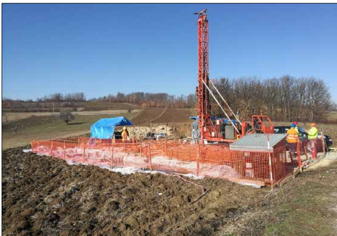
Figure 8-16: Drill rig at REK001 site in February 2020
