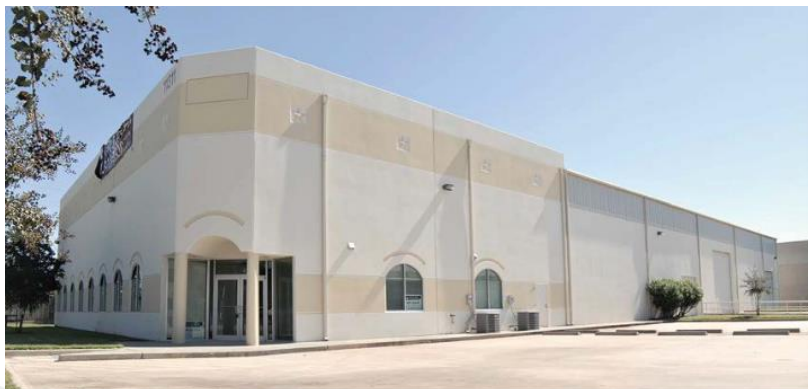
3MF's new Additive Manufacturing facility located in Houston Texas
