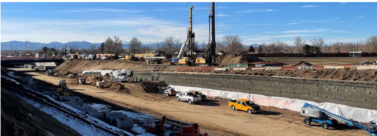
Figure 3. Shotcrete being applied on Central 70 Project
