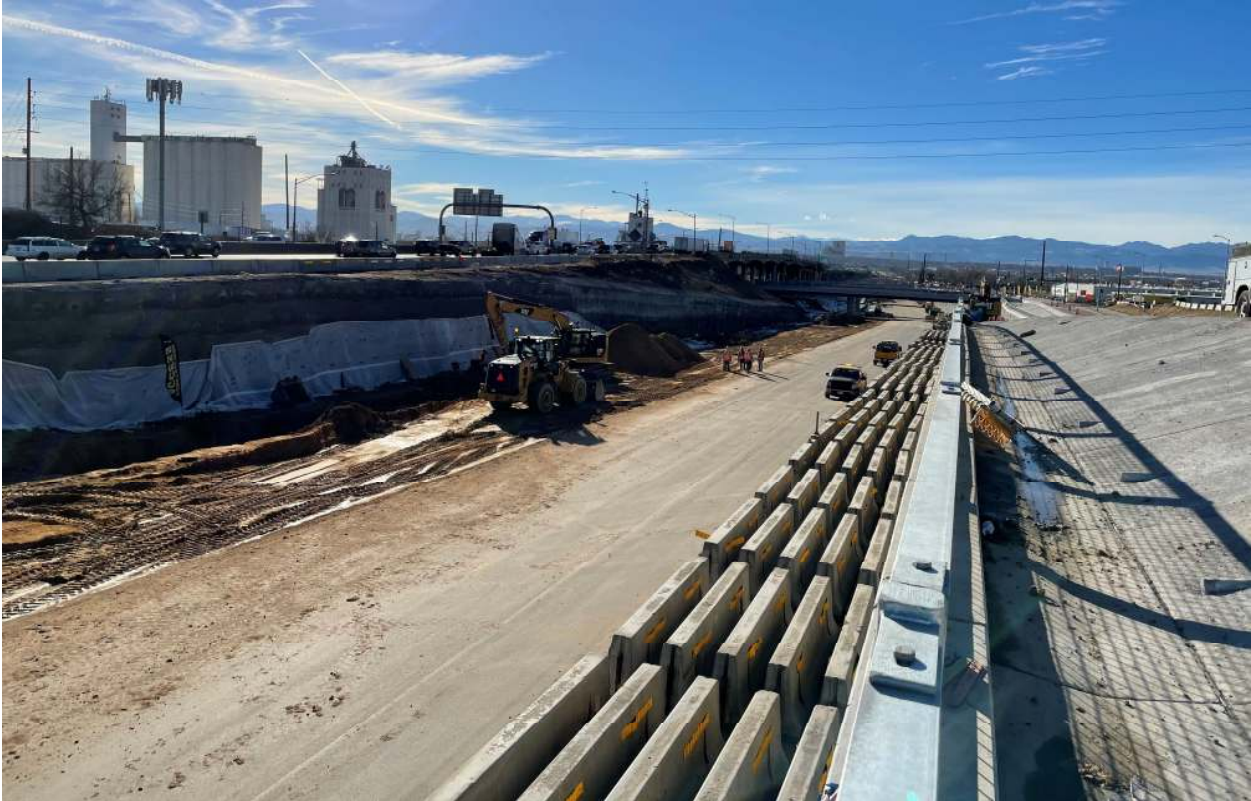
Figure 4. Section where shotcrete is being applied on Central 70 Project
