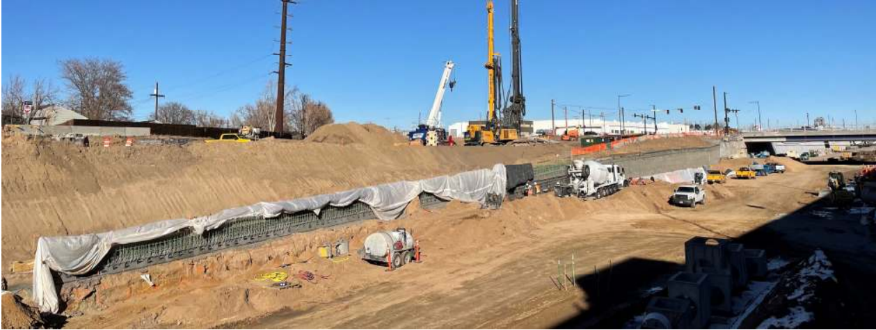
Figure 1. Shotcrete being applied on Central 70 Project
