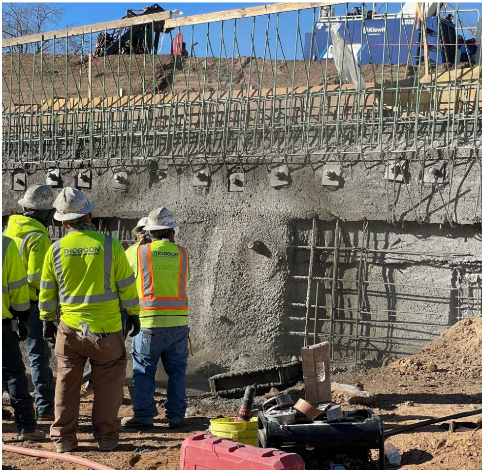
Figure 5. Shotcrete being applied on Central 70 Project
