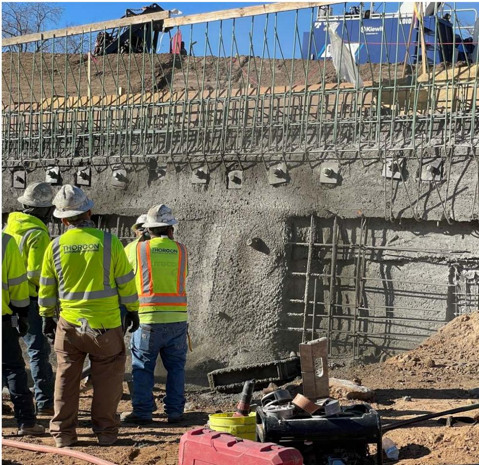
**Figure 5. Shotcrete being applied on Central 70 Project**
