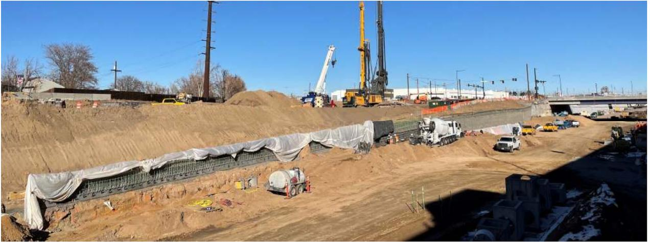
**Figure 1. Shotcrete being applied on Central 70 Project**
