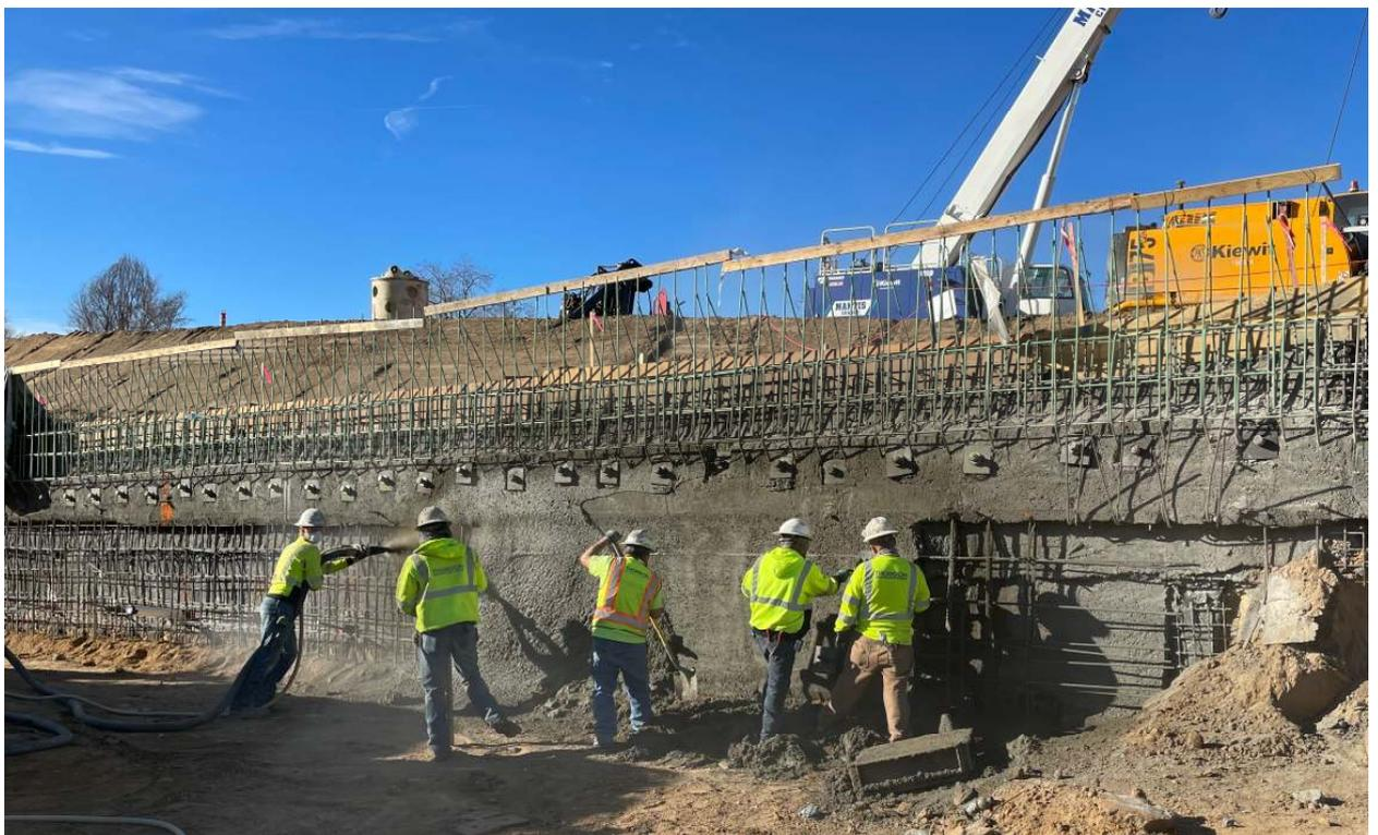
**Figure 2. Shotcrete being applied on Central 70 Project**
