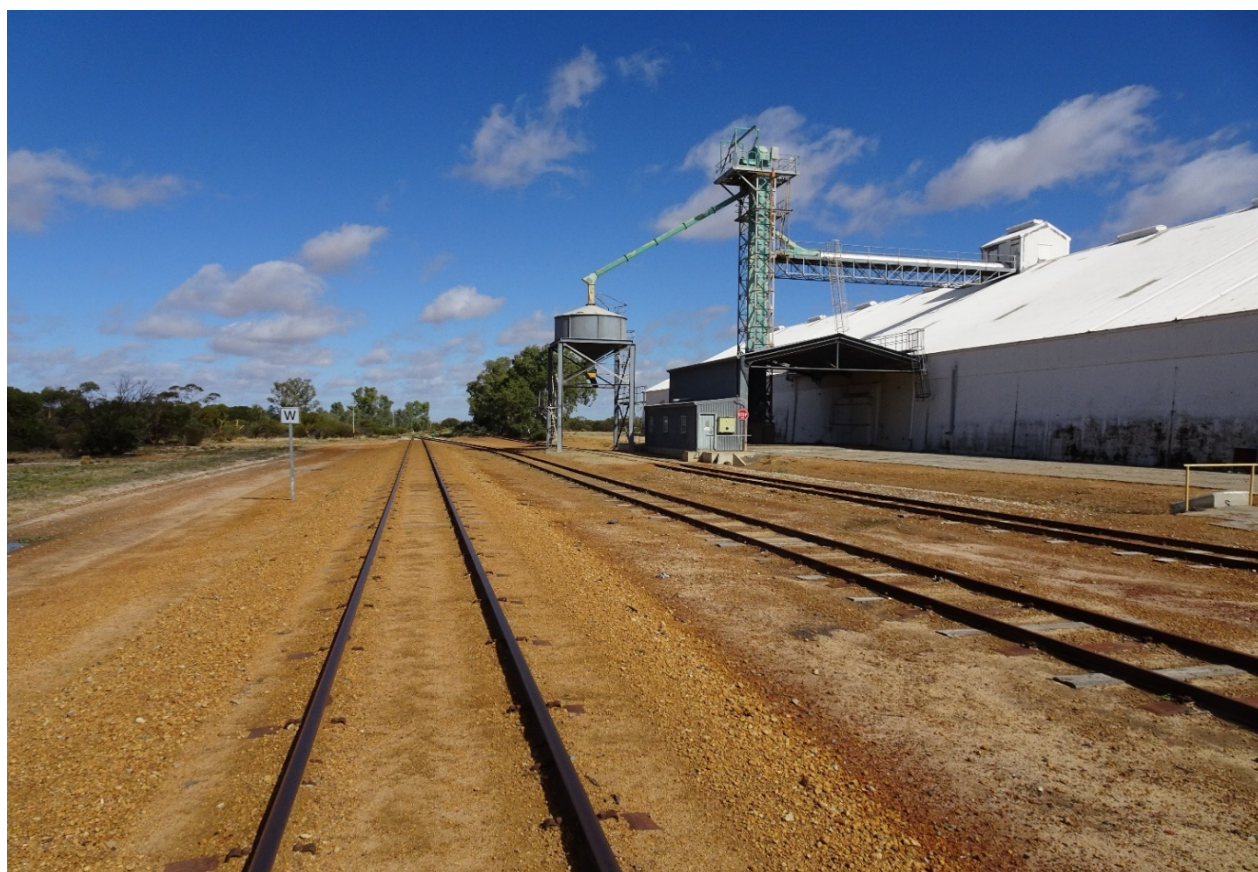
Figure 5 – CBH grain storage shed and rail siding, Gabbin, Western Australia
