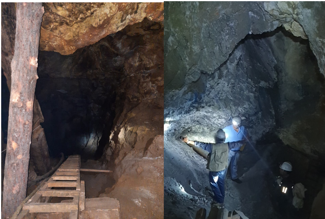
Figure 1- Cleaned out and rehabilitated underground workings
