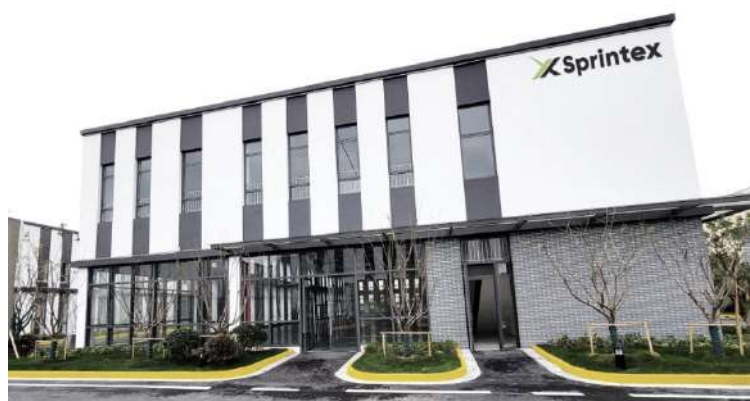
Note: Photo shows the actual building secured by Sprintex, with the Sprintex logo graphically inserted
