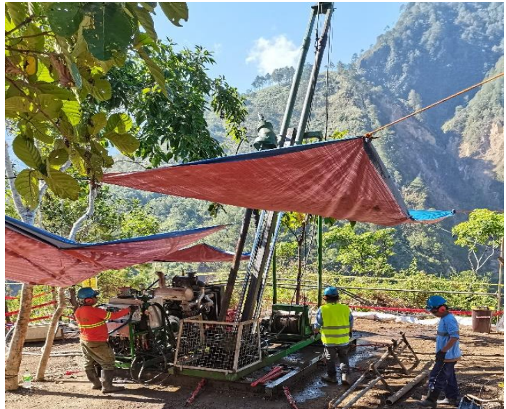
Image 2: Drill rig at MCB-034 in operation.
