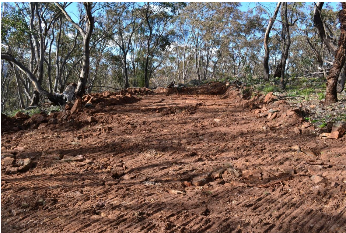
Figure 4 - Drill Pads Cleared for RC Program
