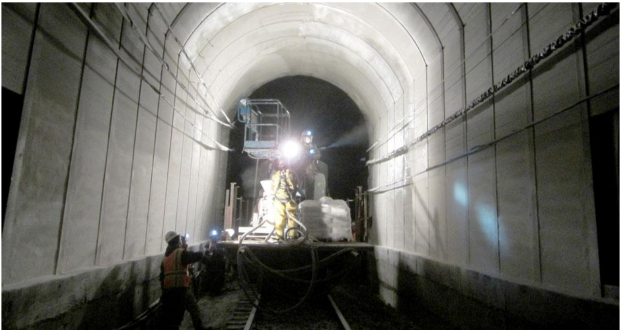
Figure 2. The interior of the Moffat Tunnel photographed during an earlier repair project (not involving EdenCrete®)
