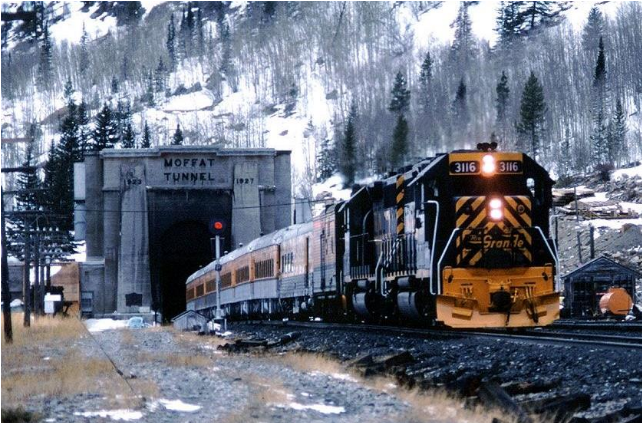
Figure 1. The East Portal of the Moffat Tunnel
