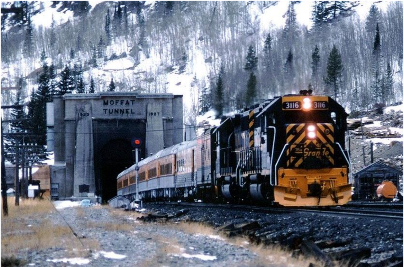
Figure 1. The East Portal of the Moffat Tunnel
