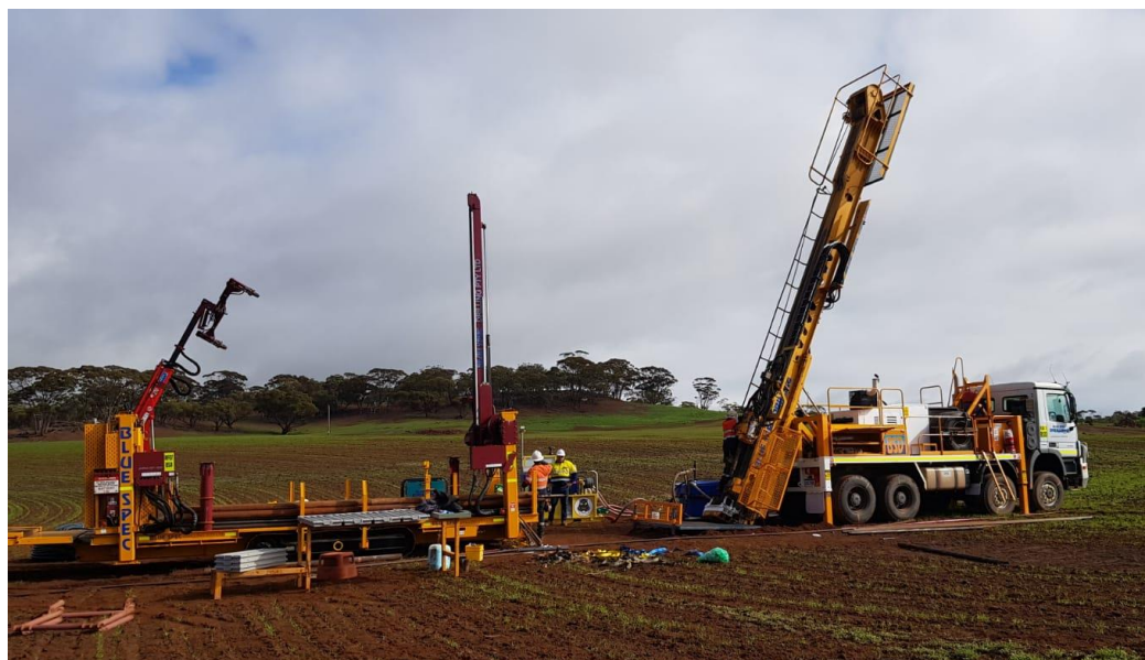
Diamond Drilling Rig at MNEWDD01
