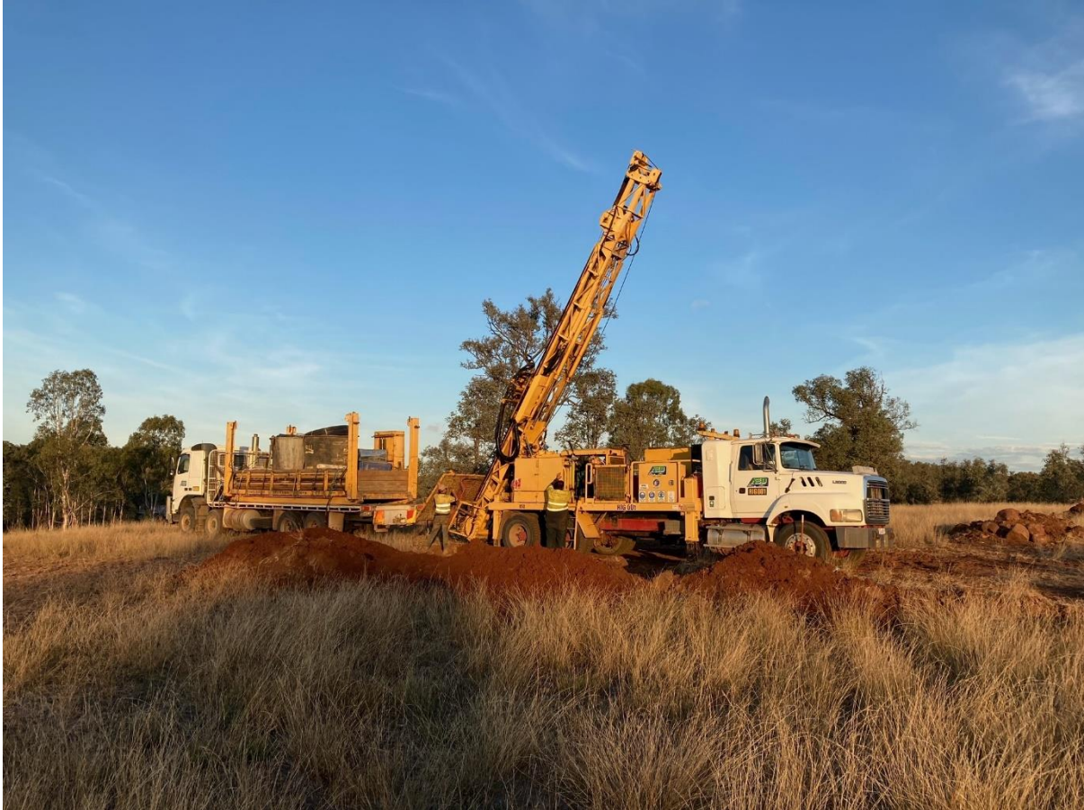
Figure 1: Diamond Rig mobilised at the May Queen gold project
