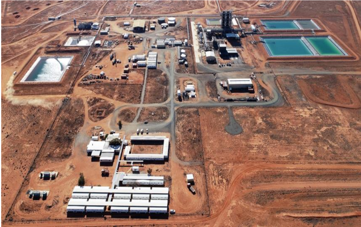
Figure 6: Existing Honeymoon process plant and infrastructure
