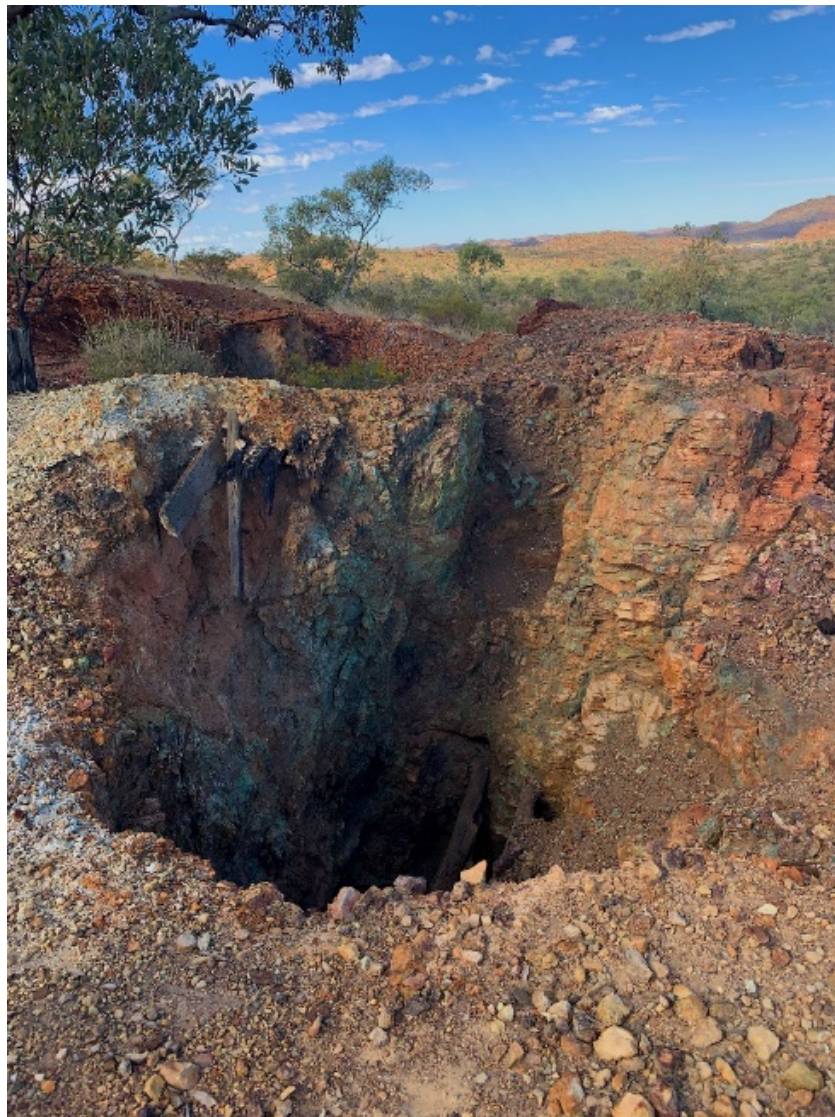
Figure 2. Lakeview eastern shaft which records indicate is approximately 28m deep
