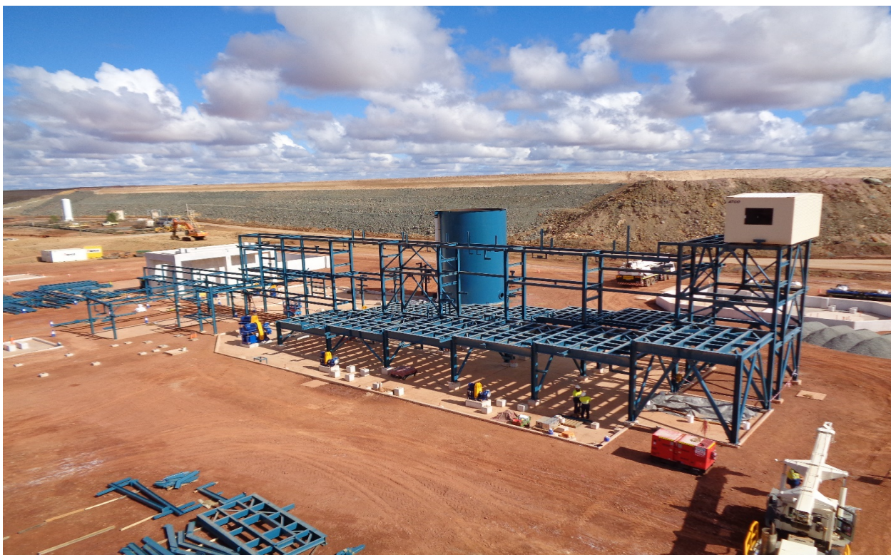
Figure 3 | Steel work to support float cells
