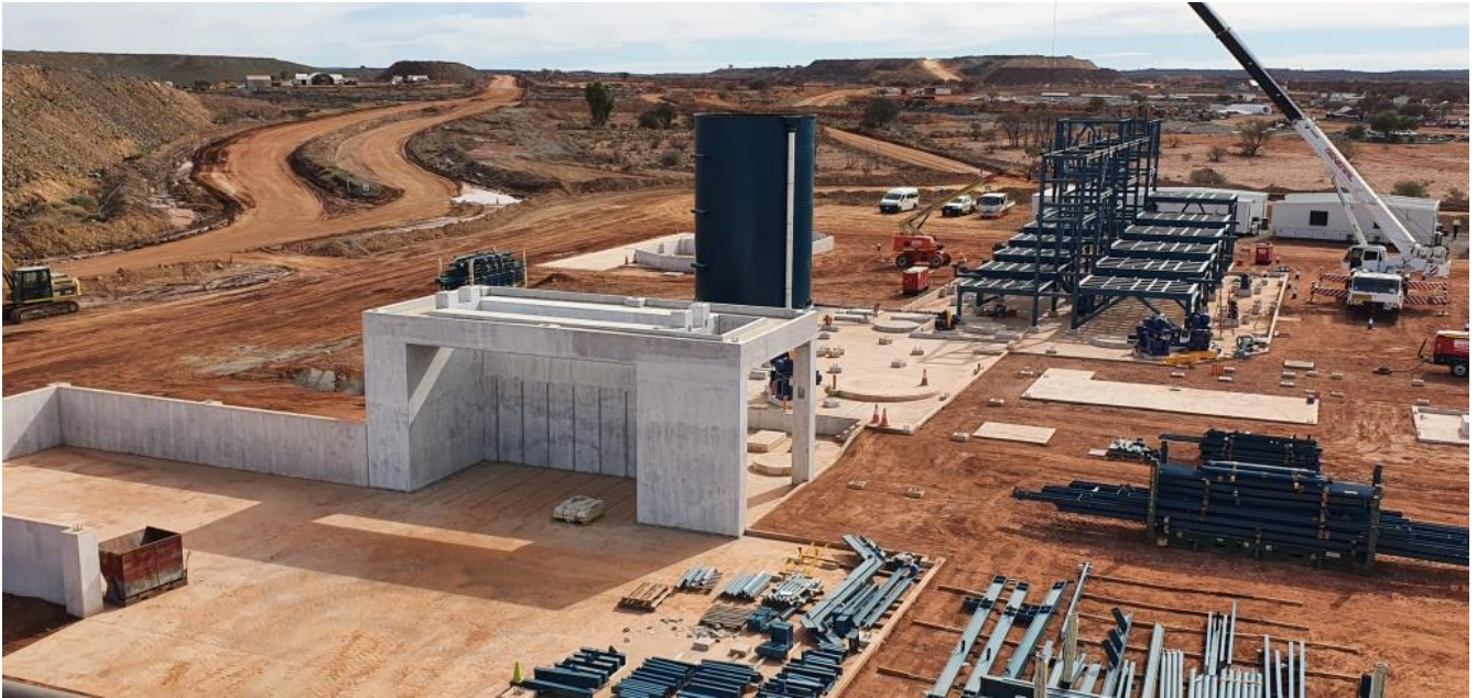
Figure 4 | Filter Building and Concentrate Storage Shed floor
