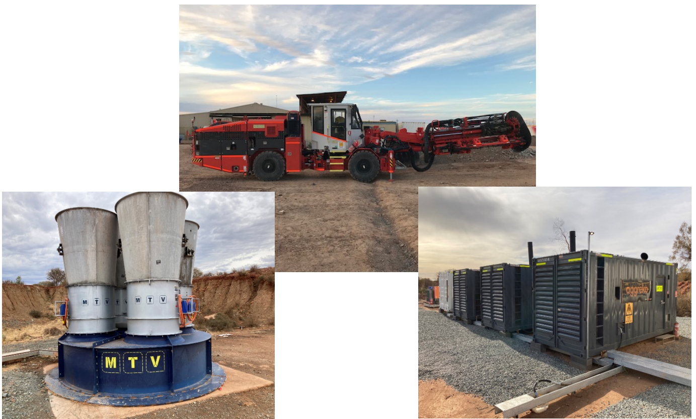
Caption | Underground Mine Development – new infrastructure and equipment
