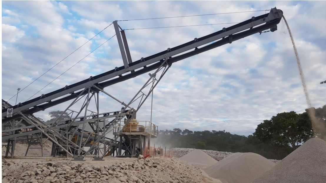
Figure 1 – Operation of the Crushing Circuit
