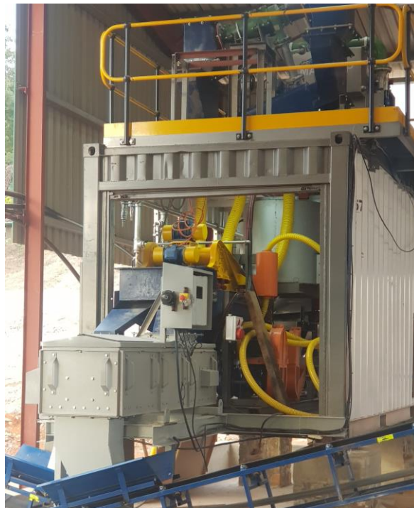
Figure 2 – Commissioning of the DMS Module in position within DMS Shed
