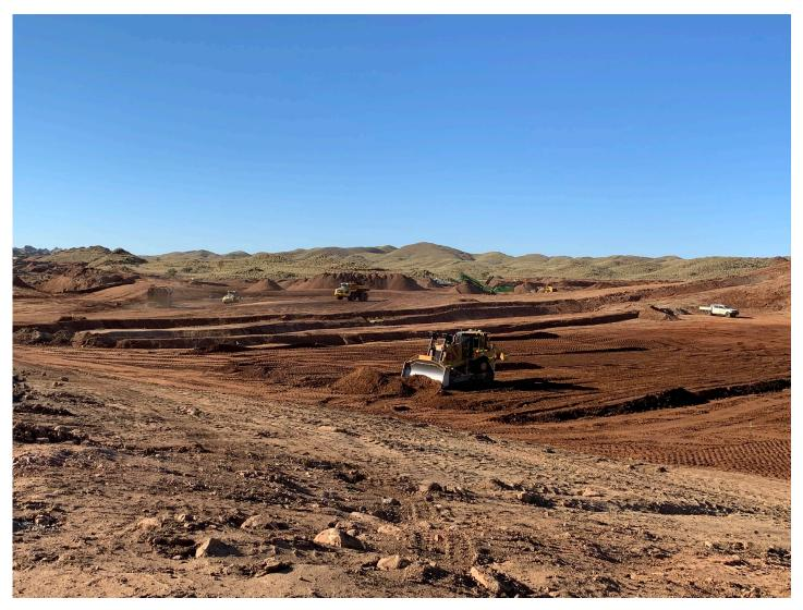
Figure 5: Tails Dam foundation preparation
