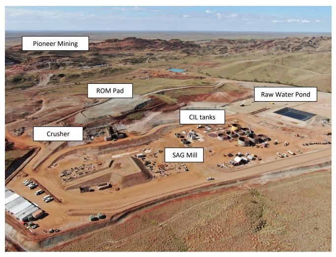
Figure 1: Processing Plant Area looking North-East
