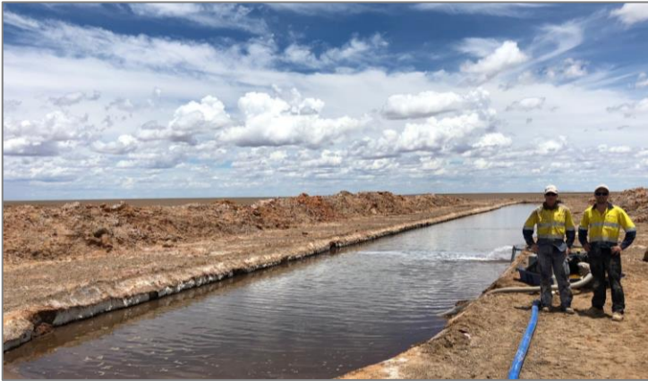
Shallow Water Table for Trench Brine Extraction
