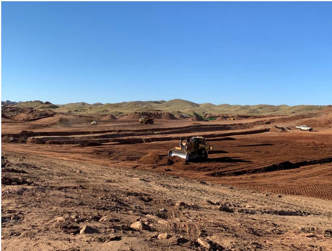
Figure 6: Tails Dam foundation preparation
