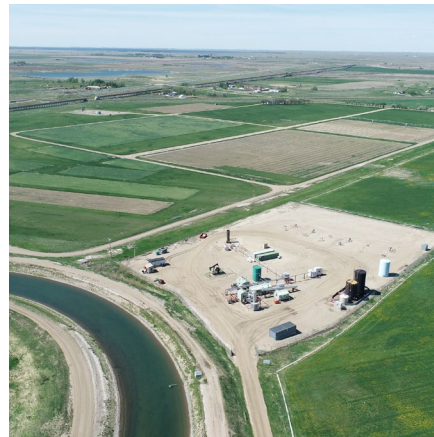
➤ Bantry 15-23 oil battery and Sunburst well pad
