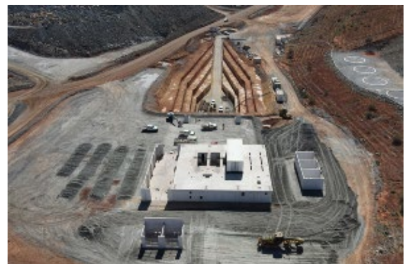
Final earthworks under way
