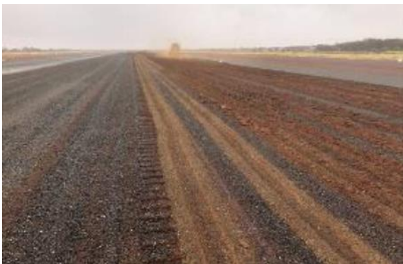
Aerodrome runway seal removal
