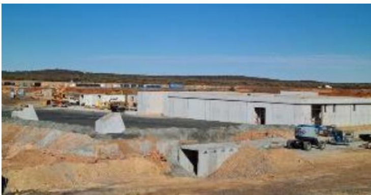
Winder house and raker leg foundations and services culverts complete
