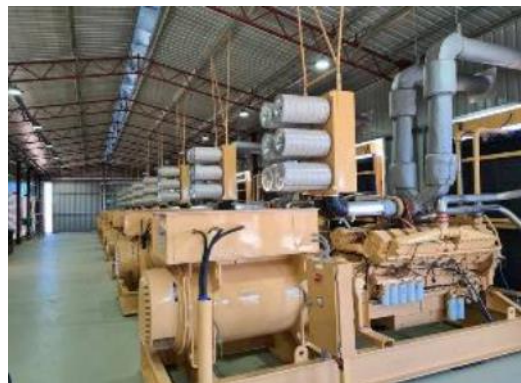
Temporary power station commissioned
