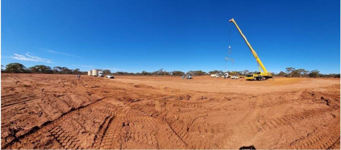
Preliminary Site works and delivery of tanks
