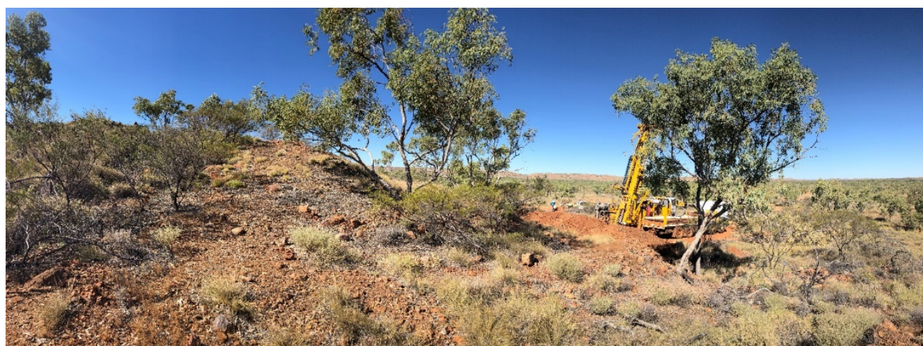
Figure 5. Rig on site at HMAKRC001
