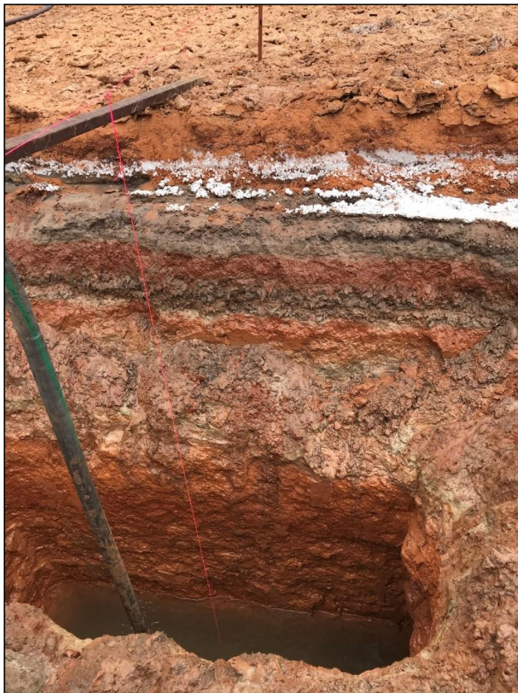
Figure 3: Test pumping of a test pit excavation
