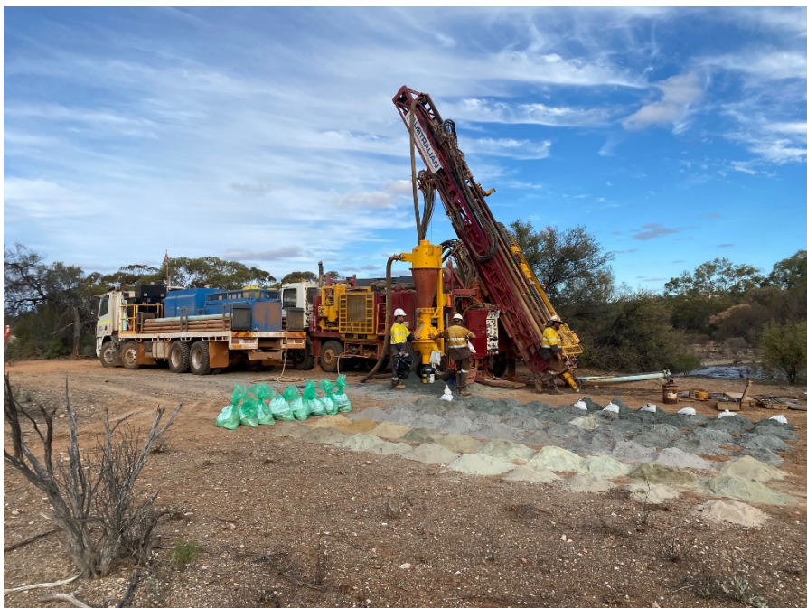
Image: RC drill rig active at the Ida Valley Project.
