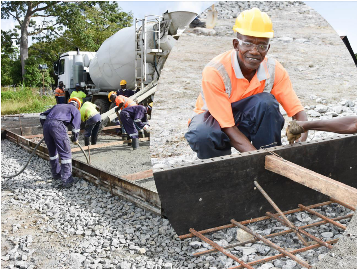
Figure 4: Concrete platforms for the 25tph plant being poured
