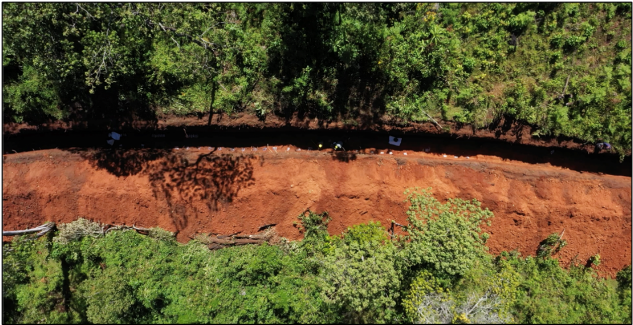
Figure 7 – Megado's team working the first trench at the Babicho Gold Project
