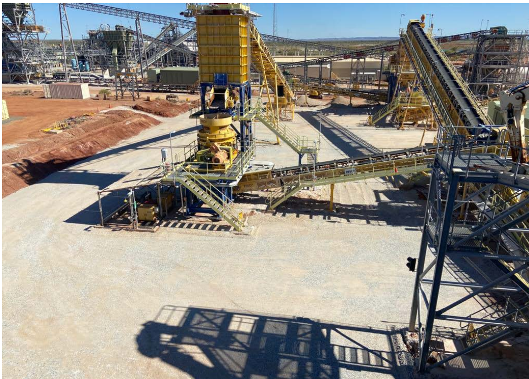
Figure 3: Completed civil works around the Ngungaju Plant
