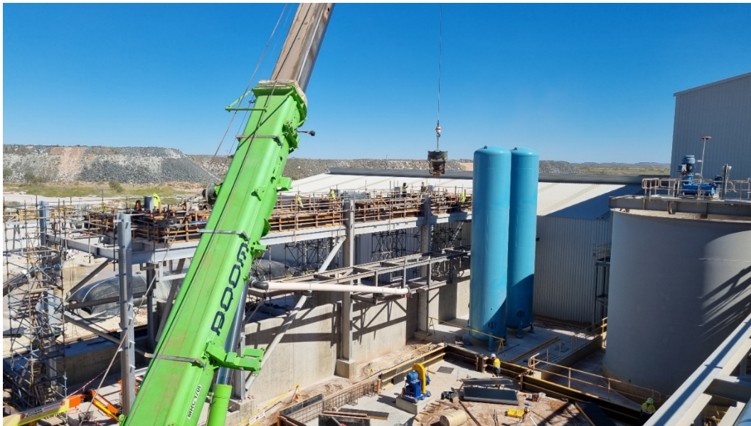
Figure 4: Installation of the filter press as part of the improvement projects package to increase production throughput for the Pilgan processing plant
