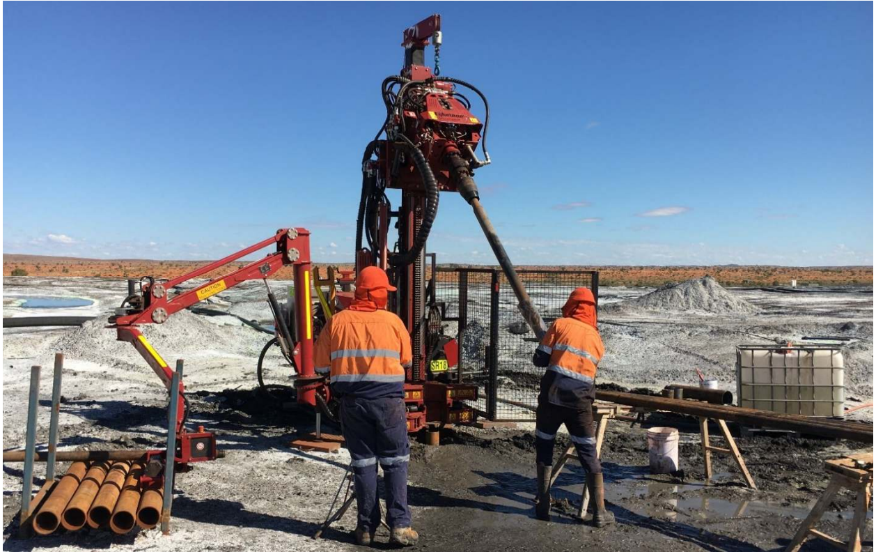
Image 1 | Sonic Rig at the Heap Leach Pads
