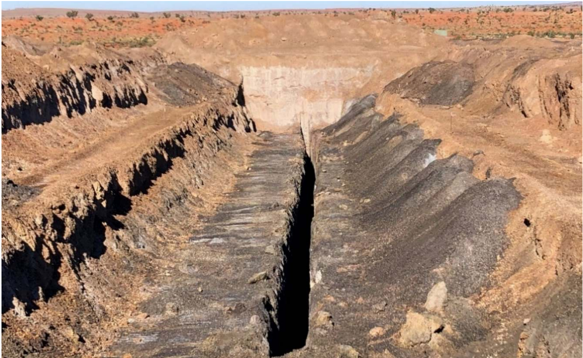
Image 4 | Trenching of the heap leach at the Nifty Copper Project
