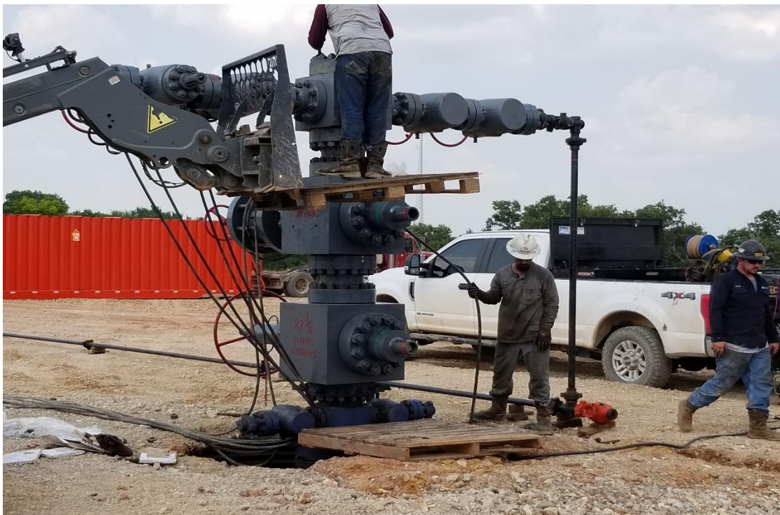
Figure 1: Installation of the completion tree on the Jewell Well.
