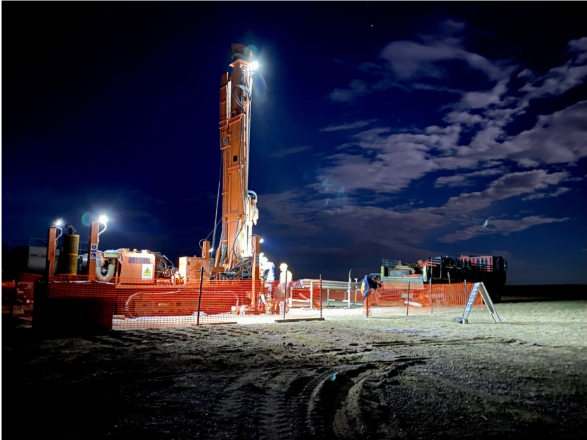
Night-time drilling in the South Gobi
