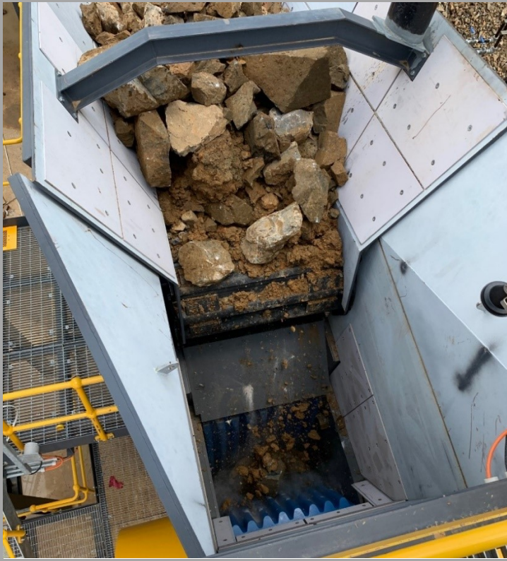
Figure 5 | Commissioning of the Jaw Crusher
