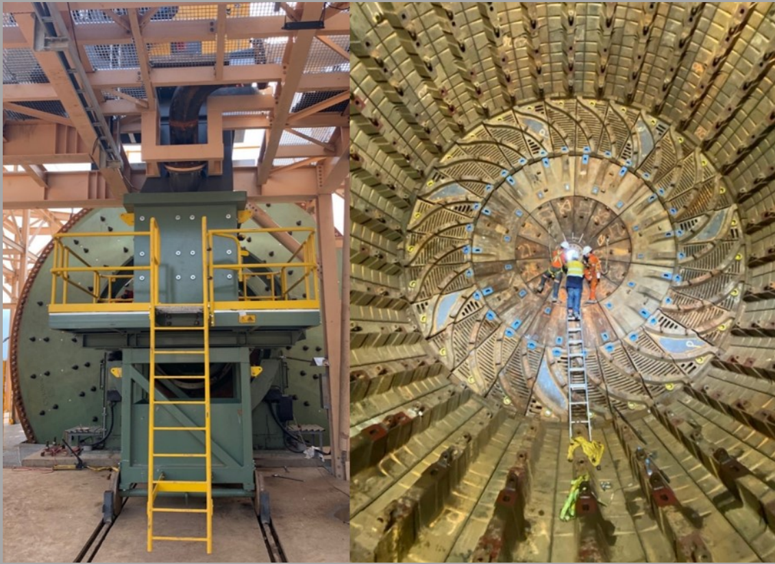
Figure 10 | SAG Mill – Commissioned and Operating
