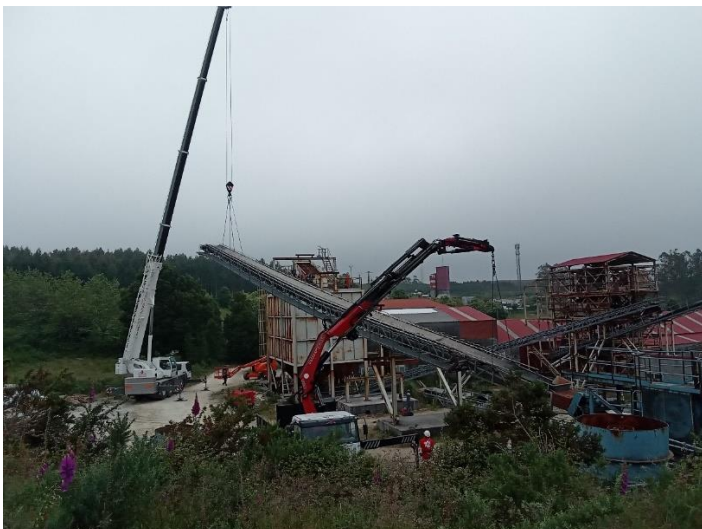
Figures 1 and 2: Dismantling and removal of the old process plant
