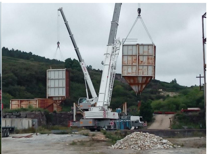
Figures 1 and 2: Dismantling and removal of the old process plant
