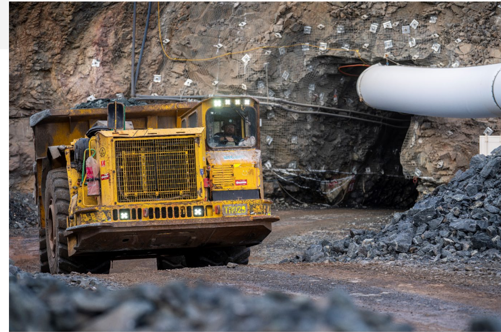
Underground portal works commenced in September 2020
