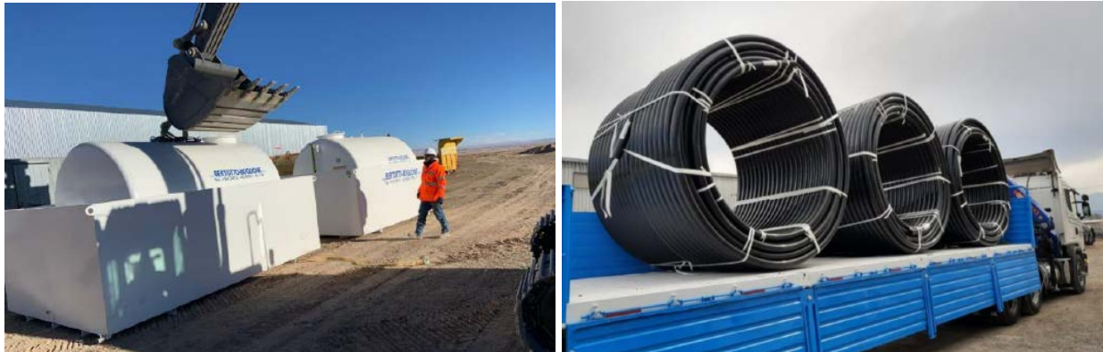
Figure 2. Rincon Lithium Project – 2,000tpa Site Operational Equipment (Site Tanks & Brine Piping)
