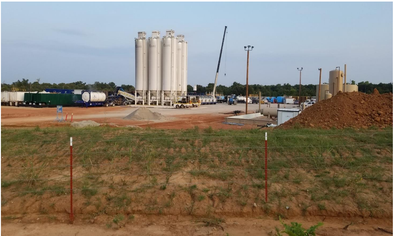
Figure 1. Liberty rigging up to commence completion operations.
