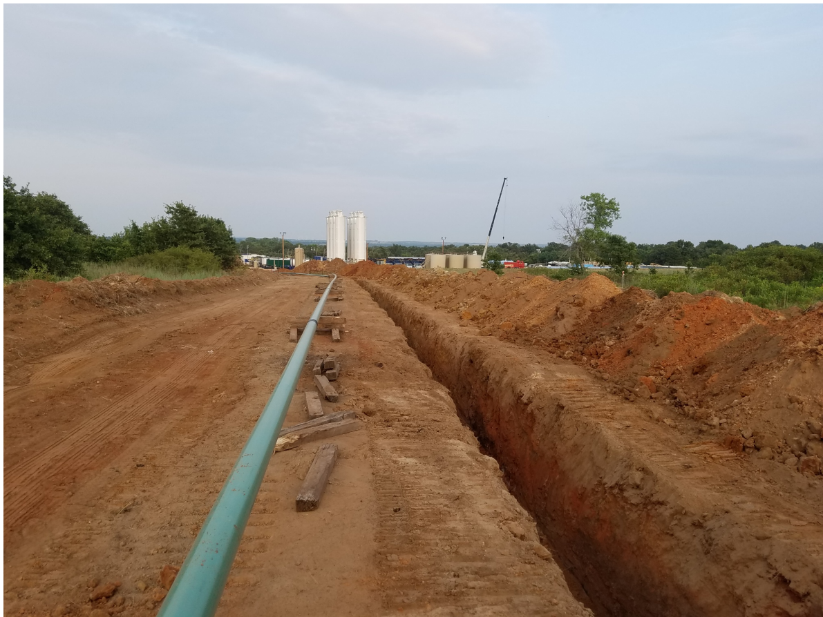
Figure 2: Gas pipeline construction from the Jewell Well pad to the tie-in point on a DCP Midstream sales line.
