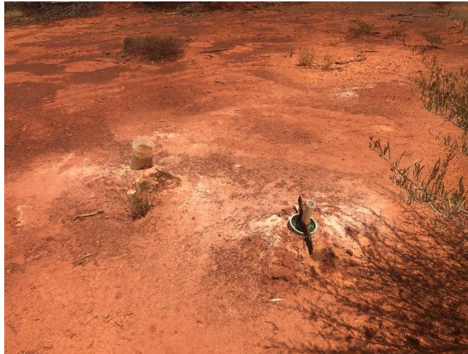
Partly Rehabilitated Drill Collars - Cannonball
