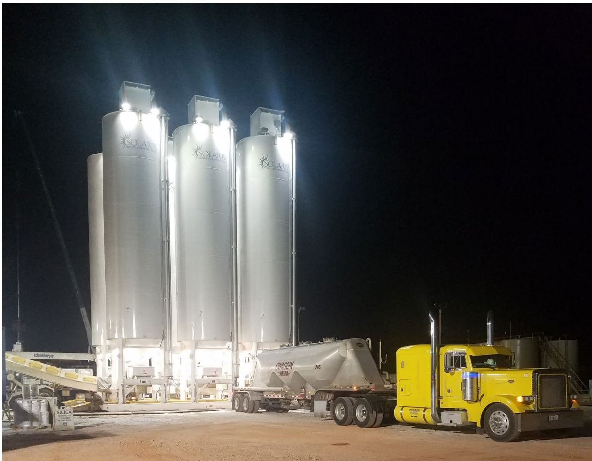
Figure 2: Delivery of completion sand to the Jewell Well site.
