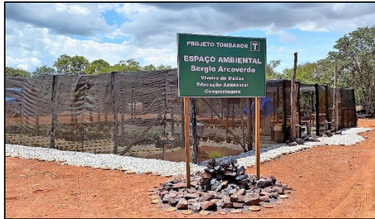
Nursery & Environmental Facility
