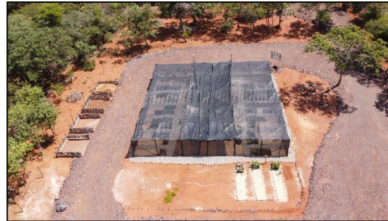
Nursery & Environmental Facility
