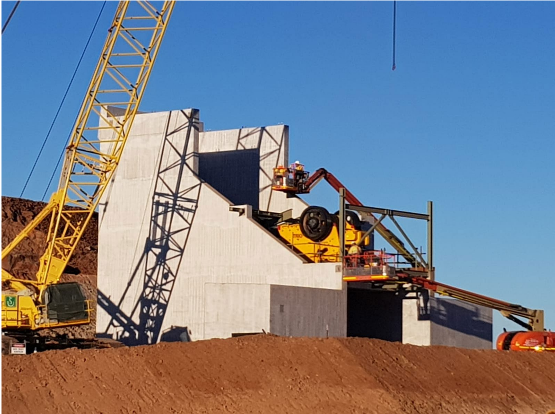
Figure 2: Crusher Installed
