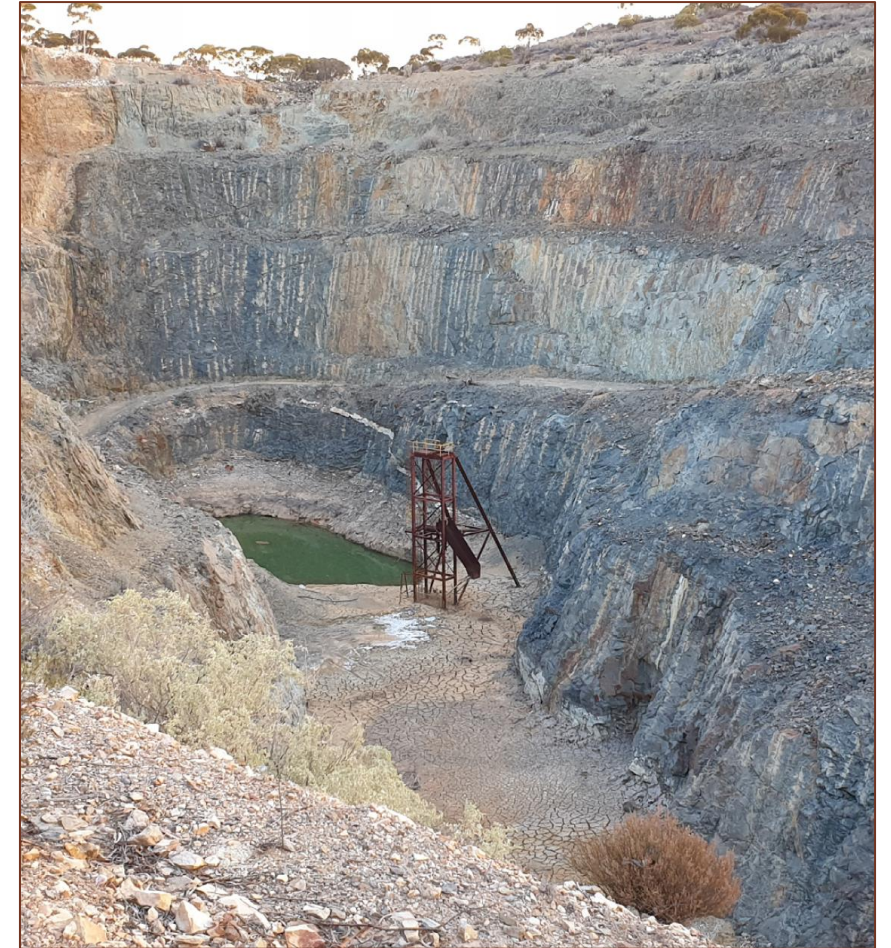
Widgie 3 Open Pit with a Shaft and remnant Mineral Resource
