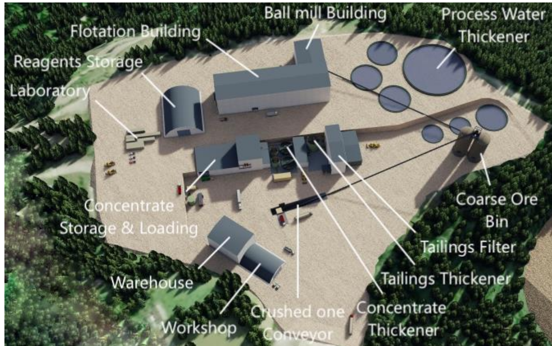
Figure 9: Isometric view of the Vares Processing Plant
