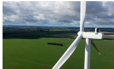
Ryan Corner Wind Farm Client: GPG Location: VIC Value: $51 million
