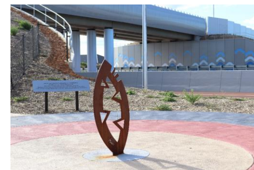
Reid Highway Widening, WA
