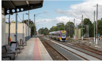
Gippsland Line Upgrade Client: Rail Projects Victoria Location: Gippsland, VIC Value: $300 million (Decmil share $120 million)
